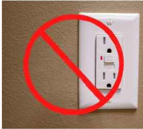
ground fault circuit interrupter (GFCI)
