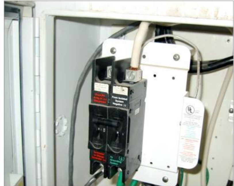
690.41(B) (GFP) Ground-Fault Protection
